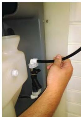
4. Connect the water supply to the inlet ball valve push-in fitting. (If you are using copper tubing, use a small section of the supplied tubing and the inline connector to connect the copper tubing to the plastic tubing. This will insure you will have a secure connection on the copper tubing away from the biocide fumes.)
