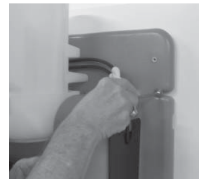
1. Drill holes for the four wall anchors with a (9/16") drill, using the mounting board as a template. Make sure the board is level. Install anchors in holes and mount the dissolver with the screws and washers provided.
