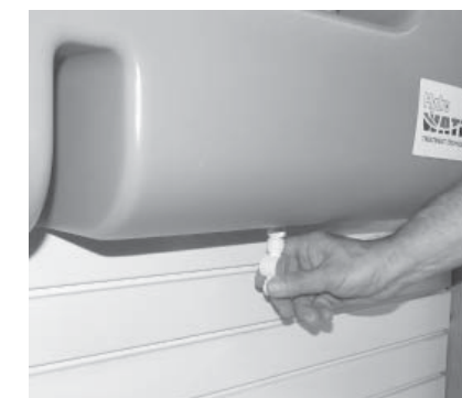
5. Install the outlet ball valve using thread sealant.
