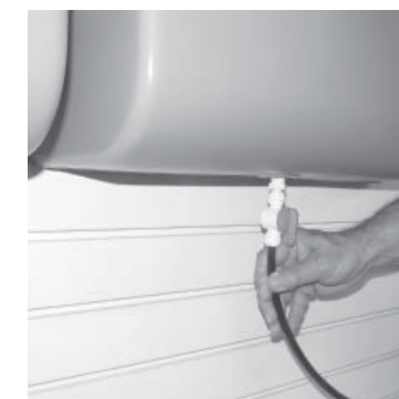
6. Connect the outlet supply line to the outlet ball valve.
