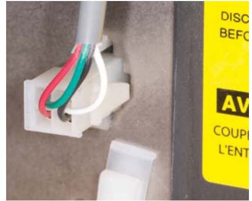
FIGURE 2: Pumpstand Flush Connector
