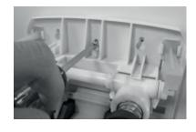
6. Place dispenser on wall bracket and install screw into the cabinet back's top center hole. **Skip to step 8**
